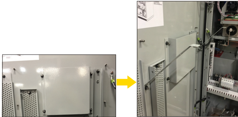
Figure 13. Location of brackets installation.
