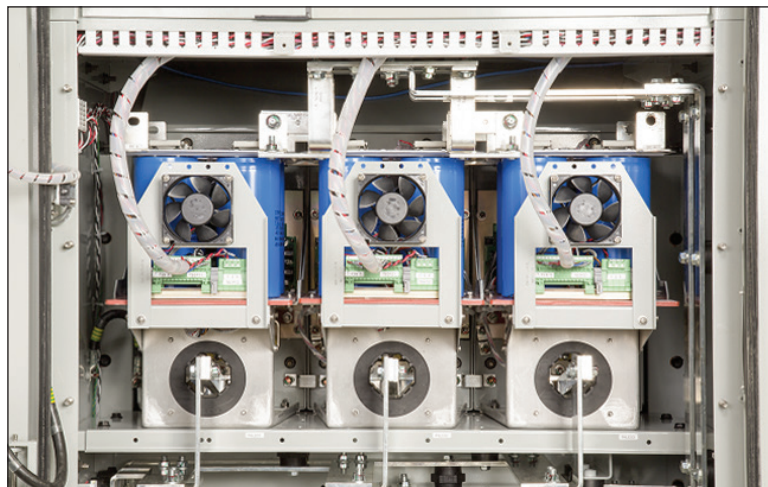
Figure 7. Inverter assembly.
