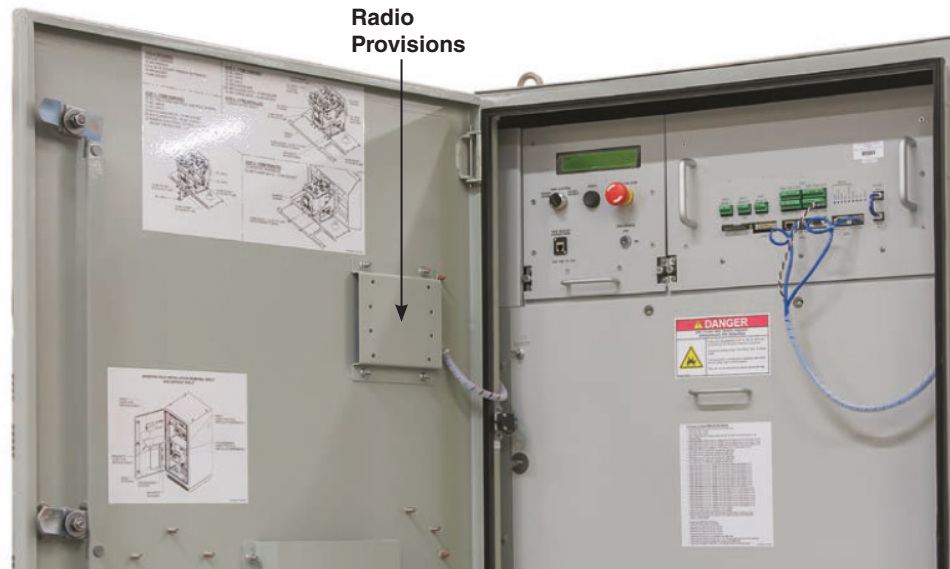
Figure 16. Provisions for radio communication.
